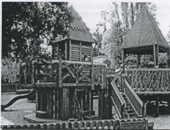
This playground in Oakland, California, designed by Leathers & Associates, is constructed with one of the new-generation preserved-wood products.
